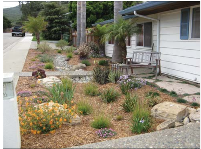
Rain garden captures and infiltrates rain water from the roof.
