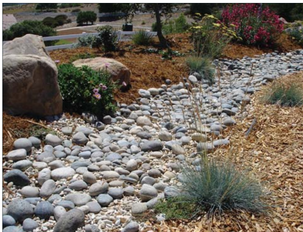
Swale infiltrates stormwater
