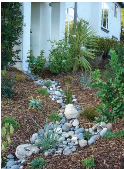
Disconnected downspout from roof of house.
