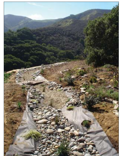
Vegetated swale under construction.
